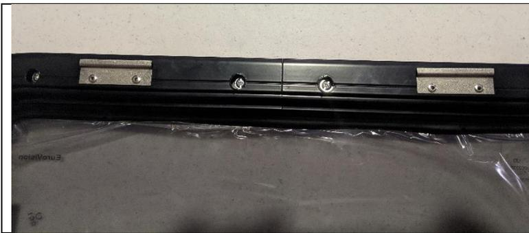
Stainless Steel lugs holding the blind assembly to the window.
