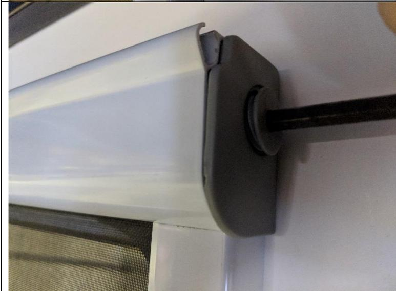
This will unscrew the larger plug and will be already putting more tension on the spring. Usually 3 to 6 turns should add sufficient tension. When enough tension is achieved, while still holding plug against container let it turn clockwise a little and the plug will lock itself back in.
