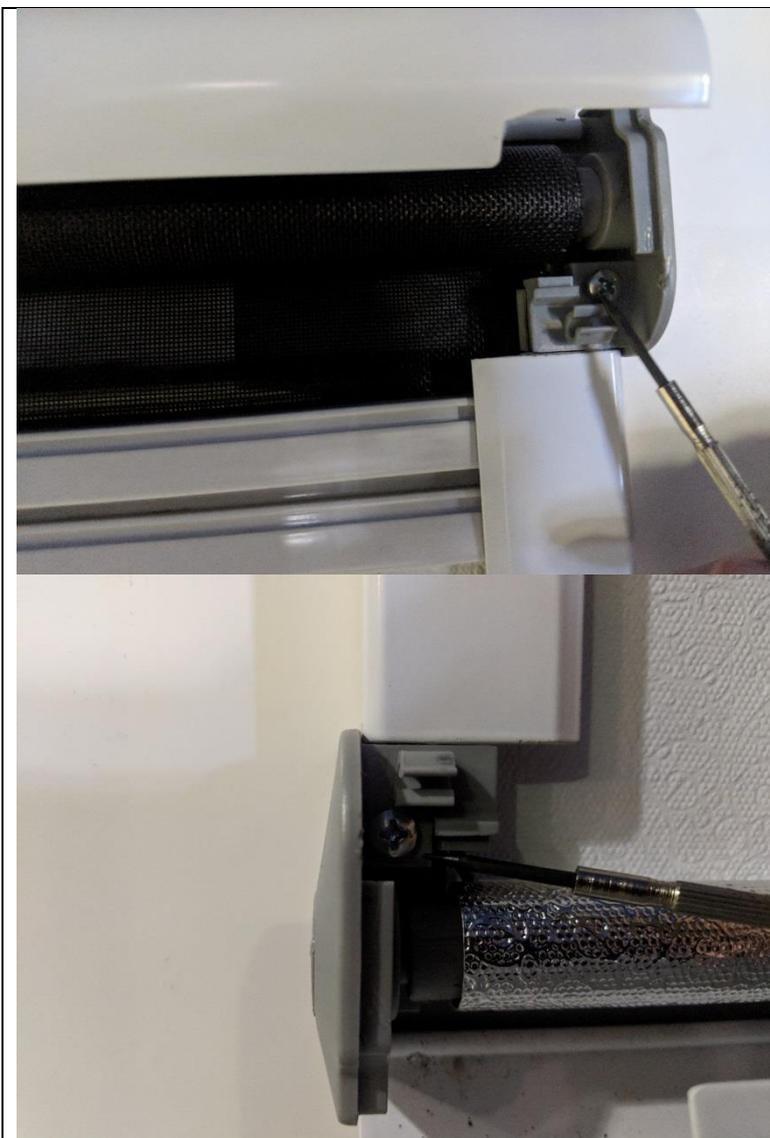
**If** blind needs to be removed due to limited space, open the container top & bottom. Remove screws from all 4 corners. Lift complete blind assembly up slightly to disengage from lugs at top of inner window frame.
