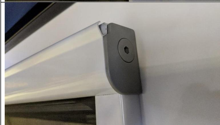
Once the plug has been removed, the 6mm hex-shaped hole should be clear.
